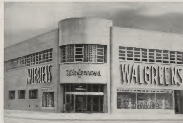
757 MICHIGAN, Chicago—Recently opened on North Michigan Avenue's "Magnificent Mile" it embodies all of our latest store design features; newest fixtures, colors, signs and other advanced construction innovations.
